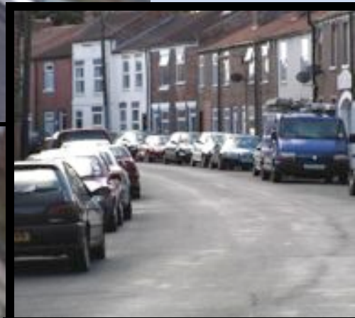
Road widening and connections
